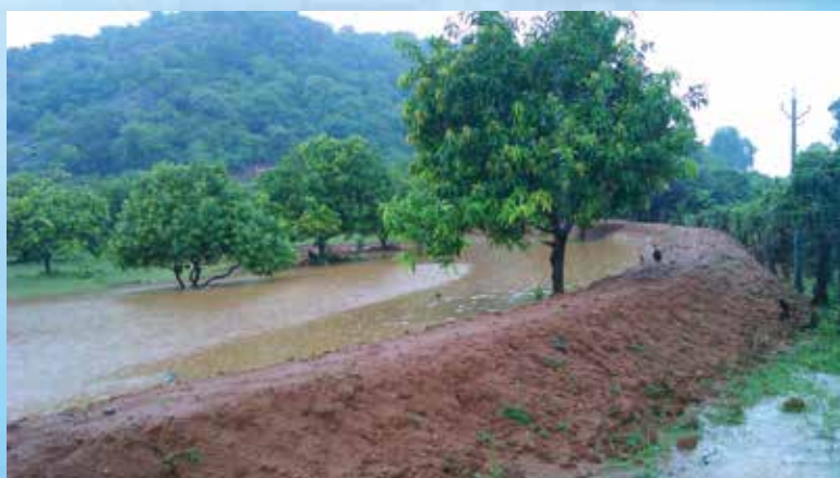
Mini percolation tank in Maddukkuru NABARD watershed
